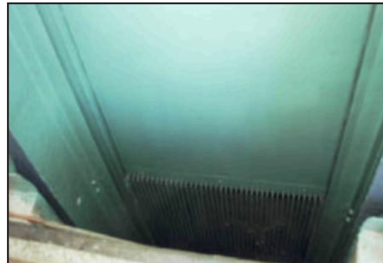
Screen frame surface after coating
