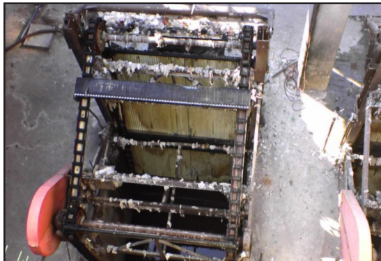
Screen in operation prior to coating
